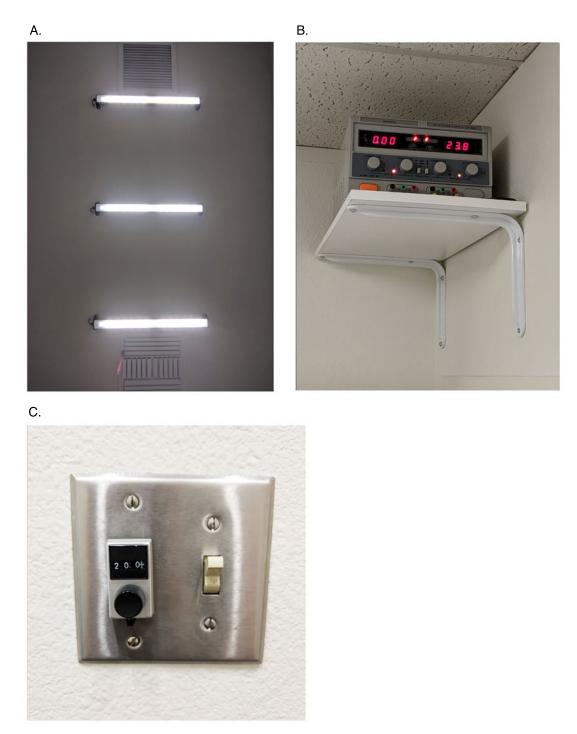
Figure 14. DC lighting set up in subject's room, including the DC-powered lights (panel A), power supply located outside testing chamber (panel B), and dimmer switch (panel C).
